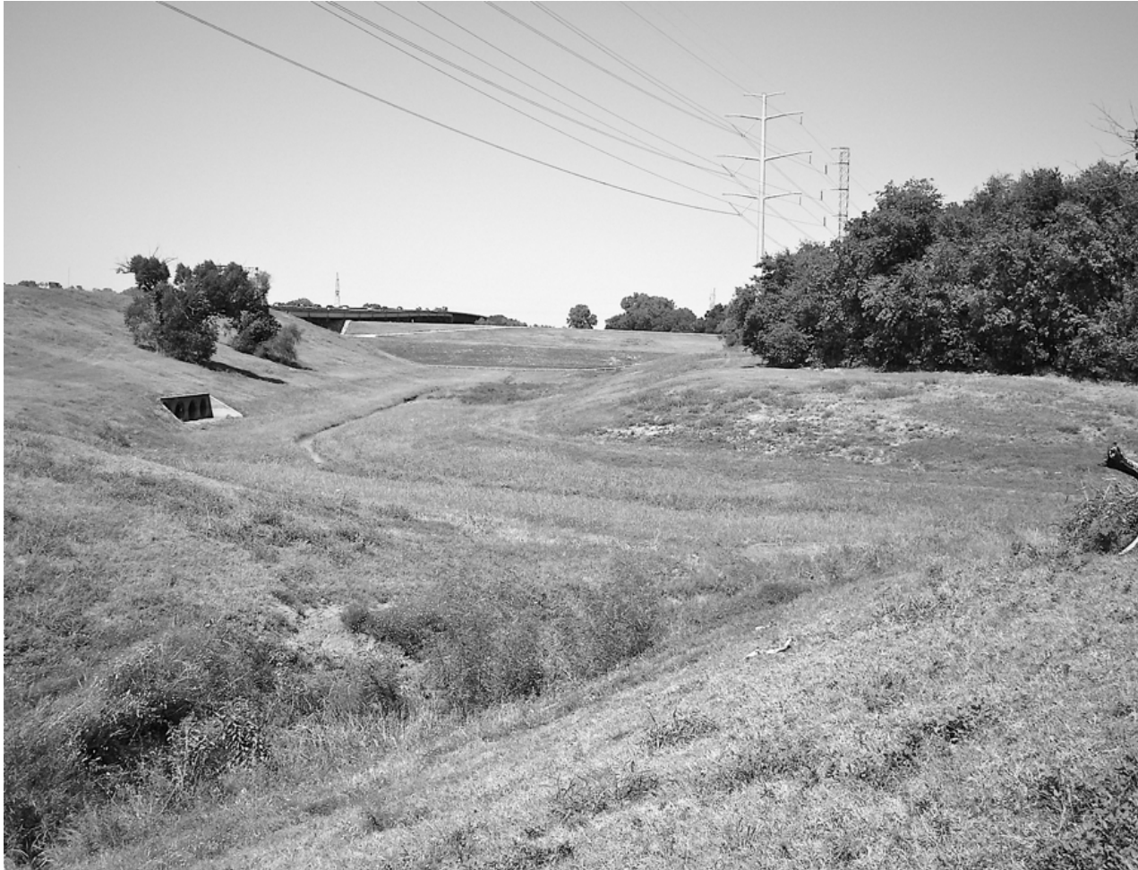
West Dallas landfill on the right with levee in the background at the intersection of S. Walton Walker (Loop 12) and Singleton boulevards, 2016. During the Superfund cleanup of the RSR lead smelter, exposed slag and battery metals at the site were covered with a 2-foot protective cap (Photo: Laray Polk).
